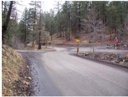
#2 Lynx Creek Bridge (end of pavement)
